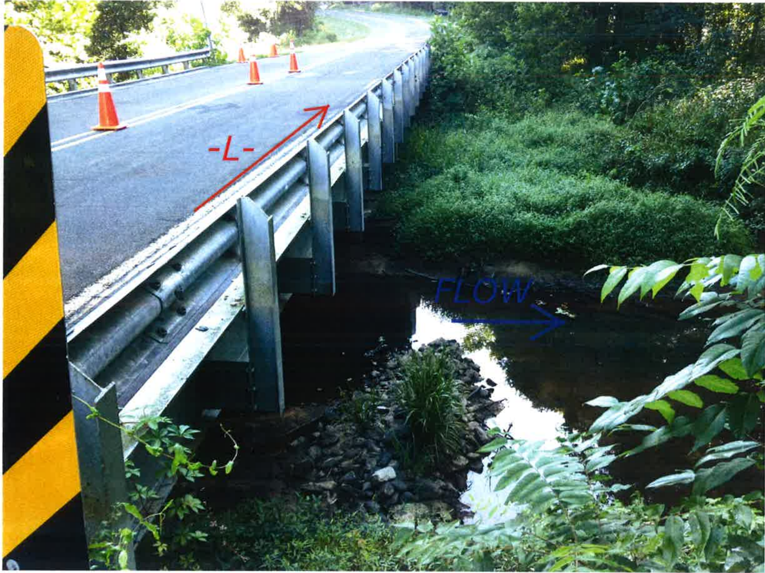
VIEW LOOKING EAST FROM END BENT 1
